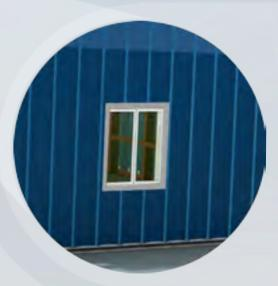
Windows Rapidset windows are available in white, bronze, or a mill finish with either single or double pane insulated glass. Windows can clip directly into an opening in the sheeting or can be framed with wall girt if requested or code dictates a low girt option.
